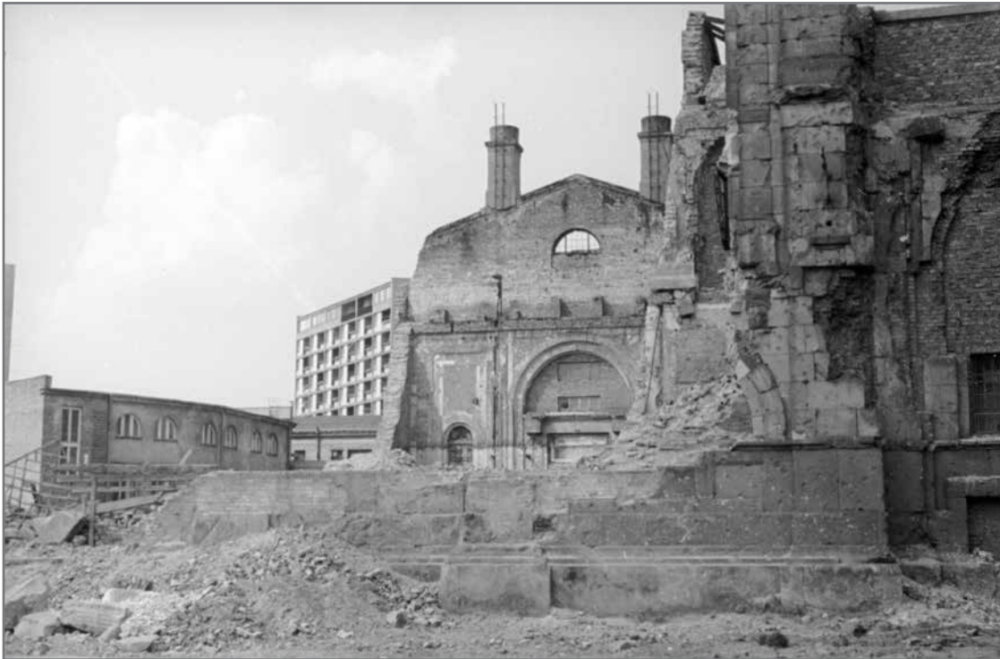
Ruins of the Bank of Poland building at 10 Bielańska St. in Warsaw, 1960s.
