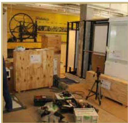
Finishing works, September – October 2015
