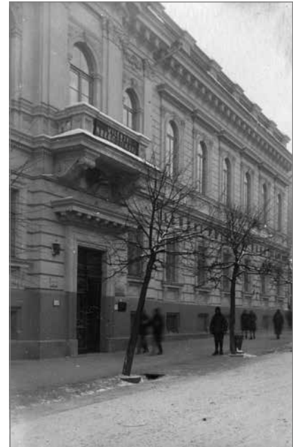
A building of the Vilnius Exchange, the interwar period, NAC Collections
